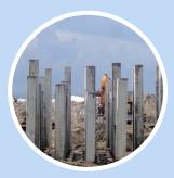
Building foundation consists of over 1,000 concrete pylons driven approximately 70 feet into the sand.
